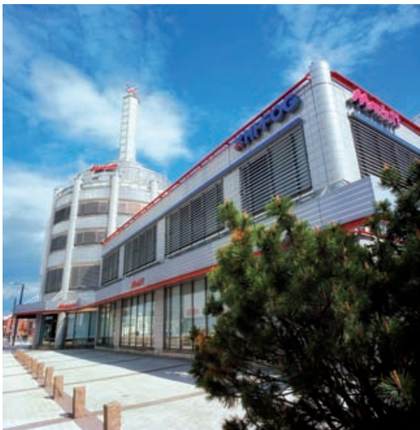
Founded in 1985, Marioff Corporation Oy has grown to become the world's leading provider of water mist systems for fire protection at sea and on land.
