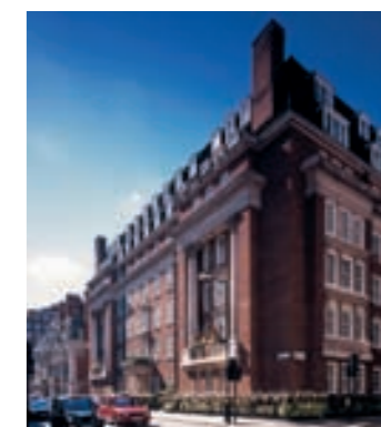
Marriott 47 Park Street Hotel, London, HI-FOG®-protected
