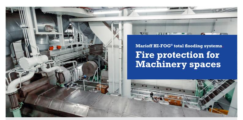
Machinery spaces, such as turbine and generator enclosures, are very susceptible to fires due to the heat generated by the equipment and the presence of highly flammable liquids. A minor malfunction or leak in machinery spaces can quickly lead to fire. The HI-FOG total flooding systems are specially designed water mist fire protection solutions for spaces like these.
