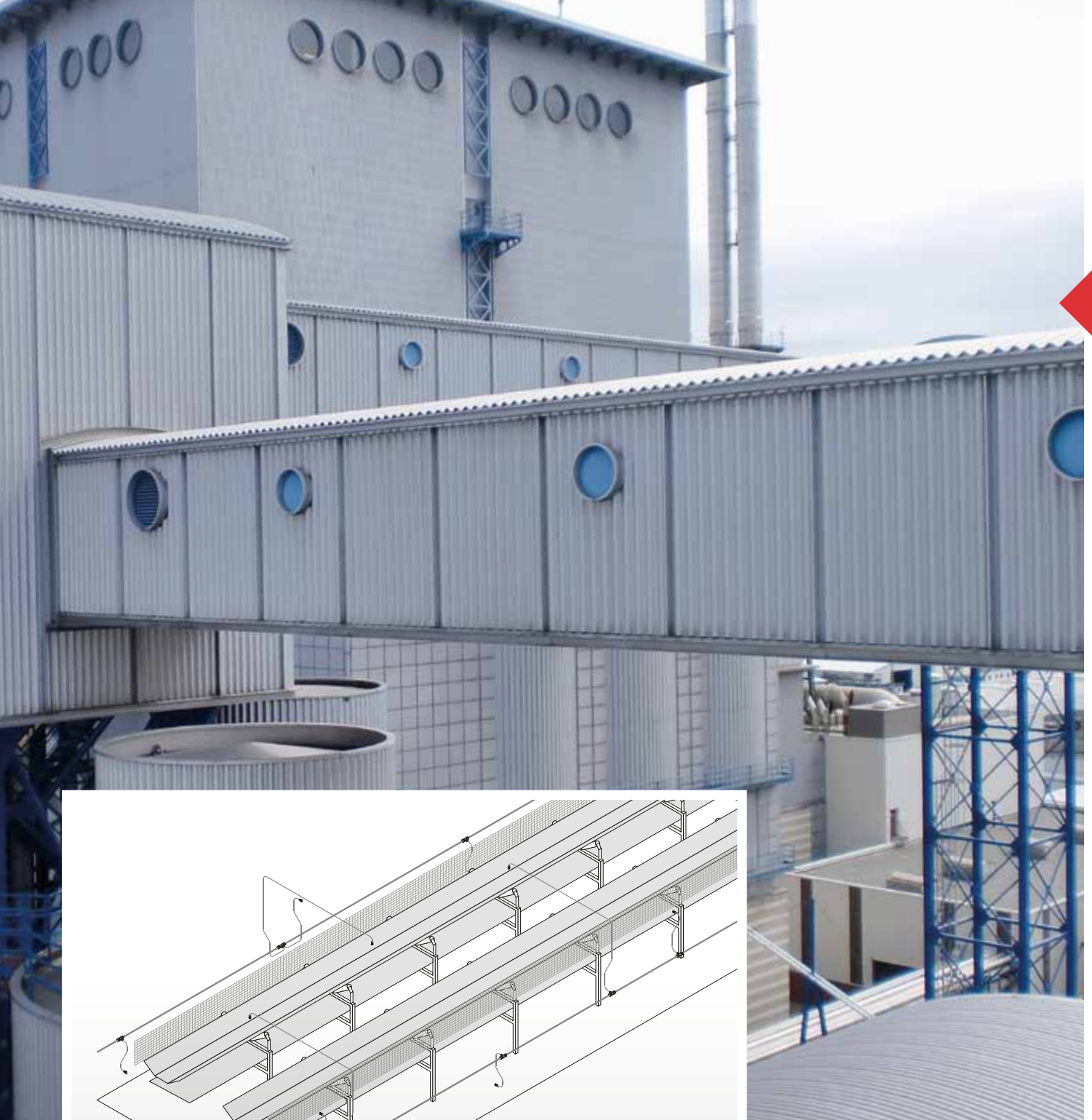
Schematic view of HI-FOG® installation for one corridor. The HI-FOG® system is also extended into the towers that join different corridors. The tubing network and nozzles run around the walls of the tower.
